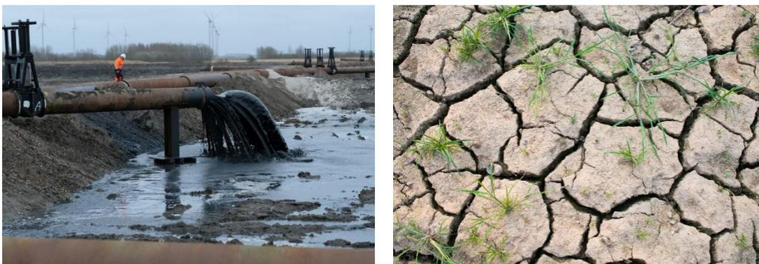
Figure 1: The start and end point of the ripening process: from fresh mud (left panel) to ripened soil with suitable mechanical properties (right panel). Photos taken from the *Kleirijperij* pilot project.
