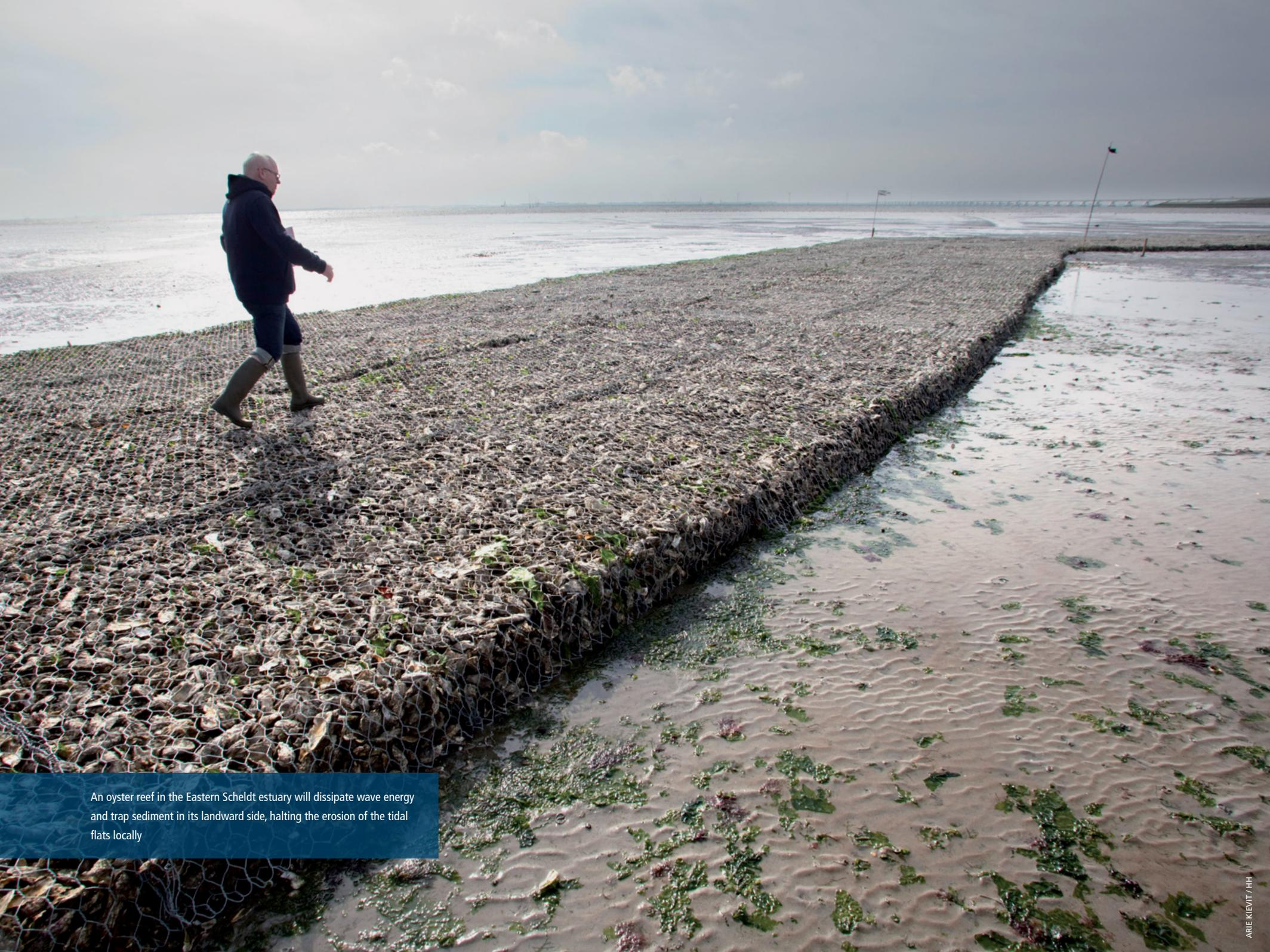
An oyster reef in the Eastern Scheldt estuary will dissipate wave energy and trap sediment in its landward side, halting the erosion of the tidal flats locally
