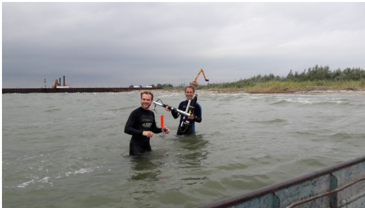
Installation of instruments for measuring the localised digging
