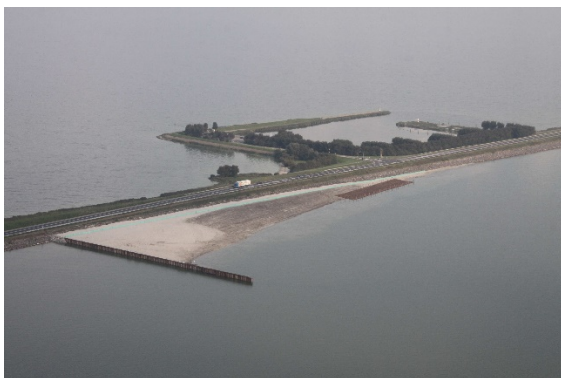
Trial section in 2014 soon after construction
