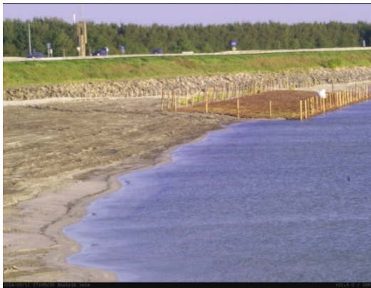
Photos made by the camera at the pilot location on 12 September 2014, with the first reeds on a braided brushwood mattress (left), and on 11 April 2015, showing a marked effect of the waves on the braided brushwood mattresses (right). Parts of the braided brushwood mattresses were washed away during the winter of 2014-2015. The planted reeds can be seen behind the mattresses.
