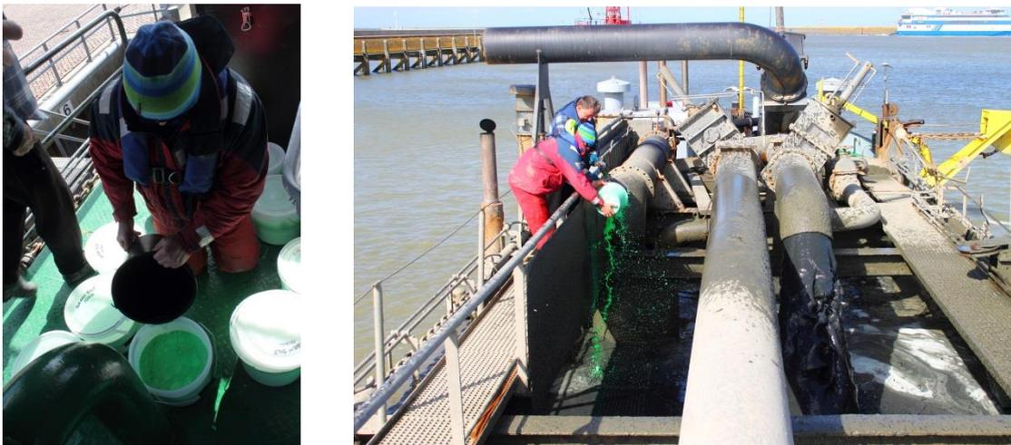
Figure 2.2 Adding water to the dry tracer material (left) and diluting the tracer with a hose while adding it to and mixing it in the hopper (right).
