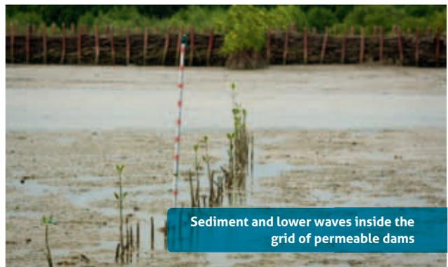
Sediment and lower waves inside the grid of permeable dams
