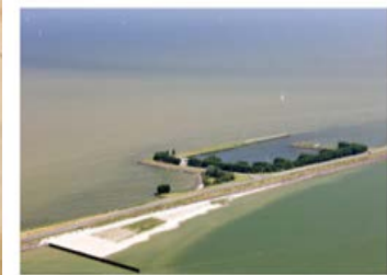
Hybrid Flood Defence Houtribdijk
