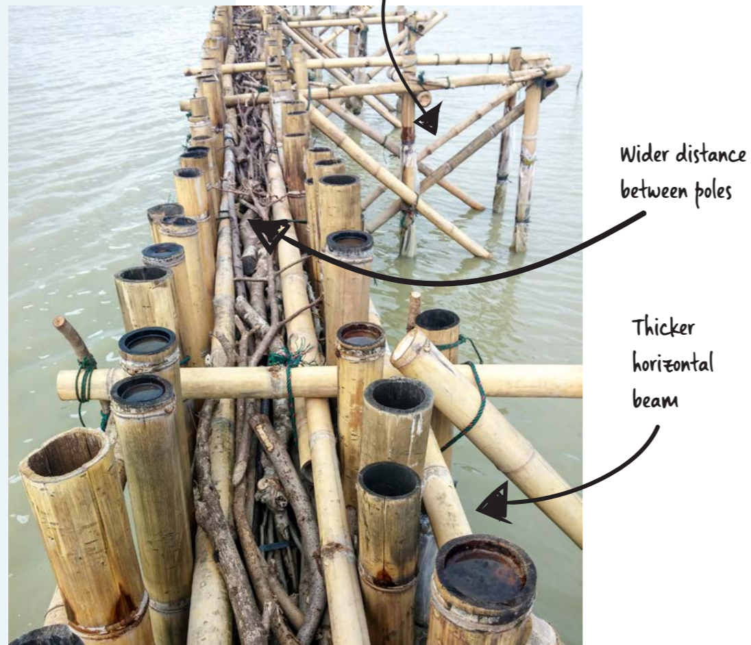
Figure 12. Alternative design that has more width between poles, support structure at the back, thicker horizontal beam © Tom Wilms, Witteveen+Bos
