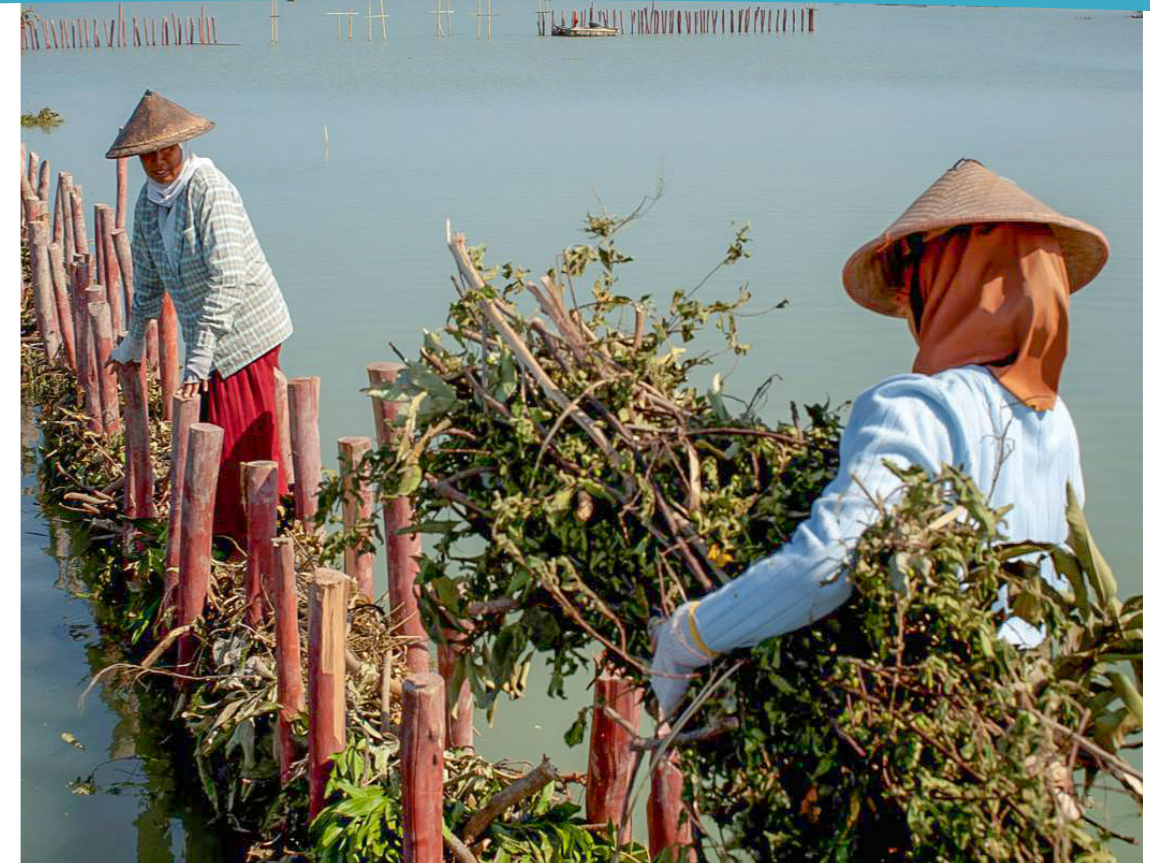
Figure 2. Construction of permeable structures by local women in Timbulloko (Demak, Indonesia) © Nanang Sujana
