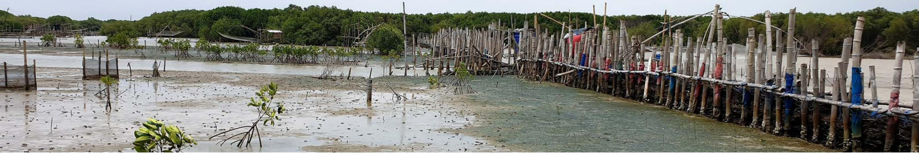
Figure 30: Increased sedimentation behind permeable structures in Demak ©Yus Rusila Noor
