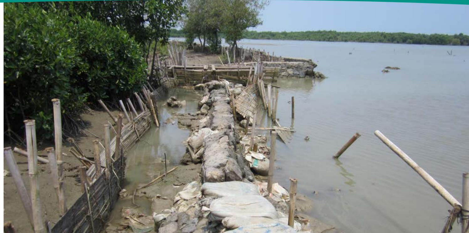
Figure 1: Failed seawall (Demak, Indonesia) © Bregje van Wesenbeeck
