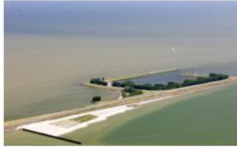
Houtrib Dike Pilot Project
